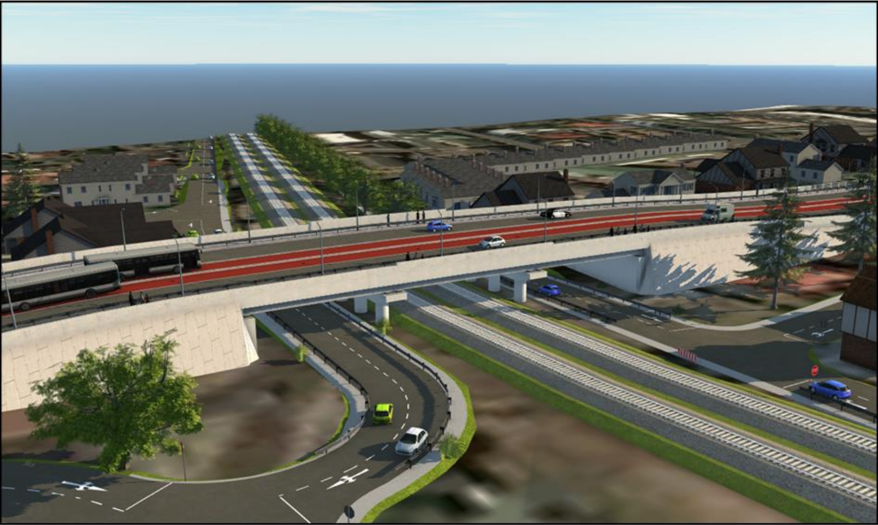
Figure 2: Conceptual view of three-span bridge (road-over-rail) (source : HHO Conceptual Design Review Report, August 2023)
