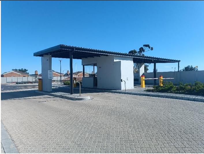
Figure 3: Security guardhouse controlling estate access
