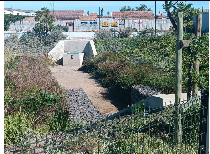
Figure 10: Condition of the stormwater attenuation pond
