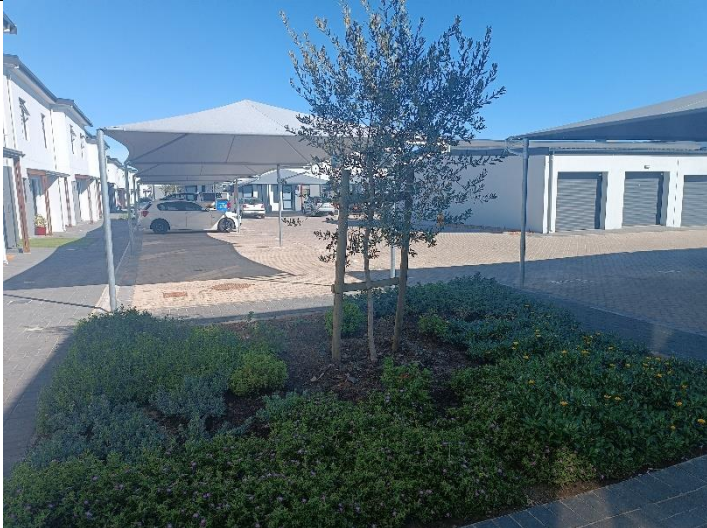
Figure 5: Landscaping which has been completed
